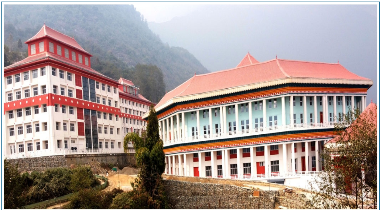
University Campus at Yangang, South Sikkim
